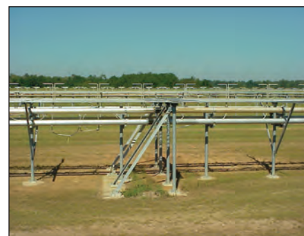
Antenna array at a NAVSPASUR station. (NRL Photo)
